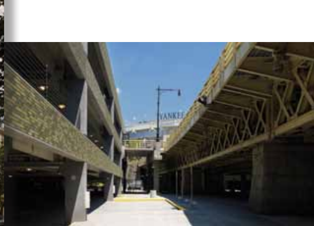
The 161st Street parking structure connects to the historic Macombs Dam Viaduct bridge, (at right), an elevated roadway 16 feet higher than the building's elevation. The garage features a continuous floor plate and an offset to provide access to the bridge's ramp.
